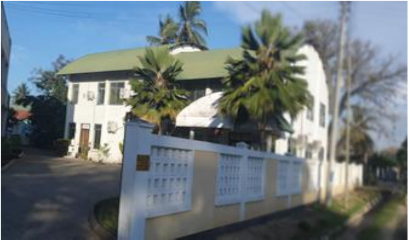
Figure 2: Bagamoyo District Council HQ
